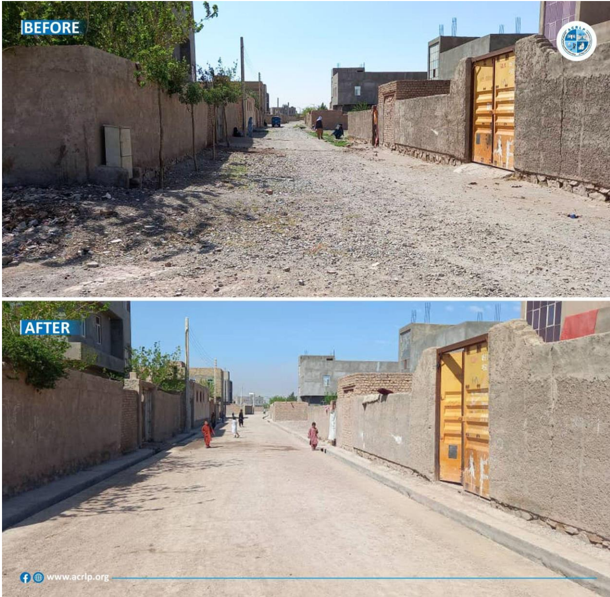
Photo. Before and after condition of gravel surface road in District 11 of Herat City on January 13, 2023
