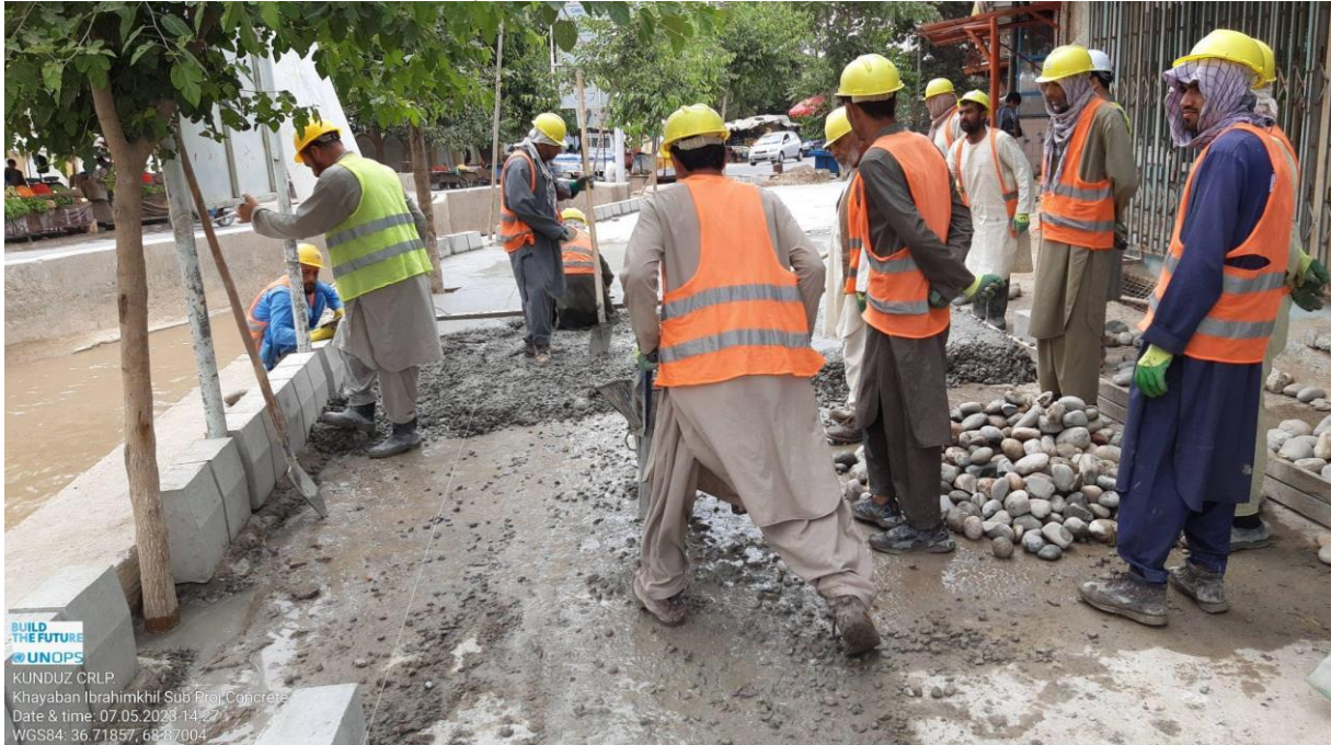
Photo: Concrete pouring process in District 1 of Kunduz Province on May 07, 2023
