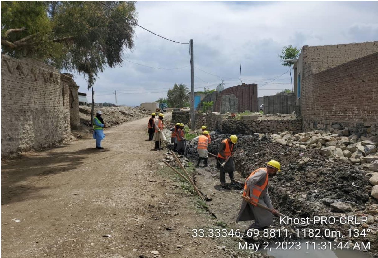
Photo: Side drainage excavation in District 6 of Khost Province on May 2, 2023
